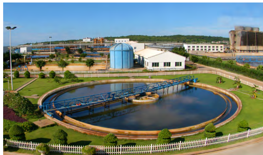
Hainan Jinhai Pulp & Paper's wastewater treatment plant
